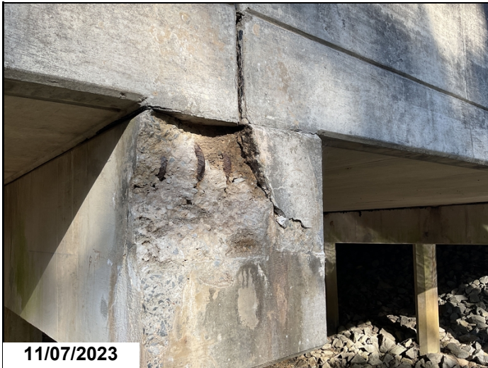
Bent 2 cap right has spall with exposed rebar.
