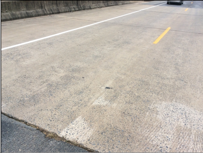
Deck - Span 1 (longitudinal crack)
