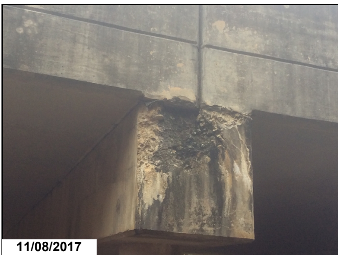
Spall at bent 2 cap on left side .
