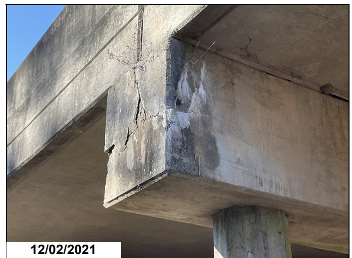
Cap - Bent 2 right: Cracking/delaminating
