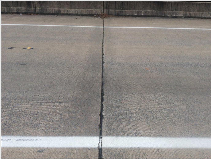
Pourable joint seal at bent 3 has loss of adhesion and debris impact, and some loss of material.
