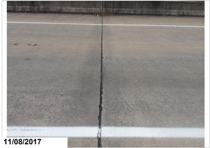
Pourable joint seal at bent 3 has loss of adhesion and debris impact, and some loss of material.
