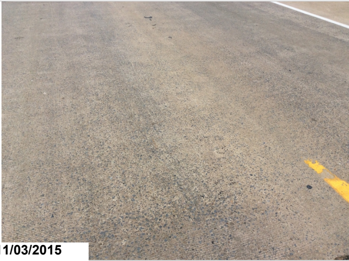
Deck - Span 2 (longitudinal crack)
