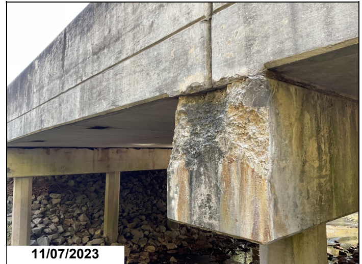
Bent 2 cap left has spalling at end.
