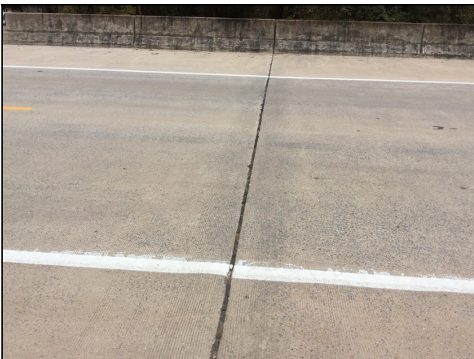
Pourable joint seal at bent 3 has loss of adhesion and debris impact, and some loss of material.
